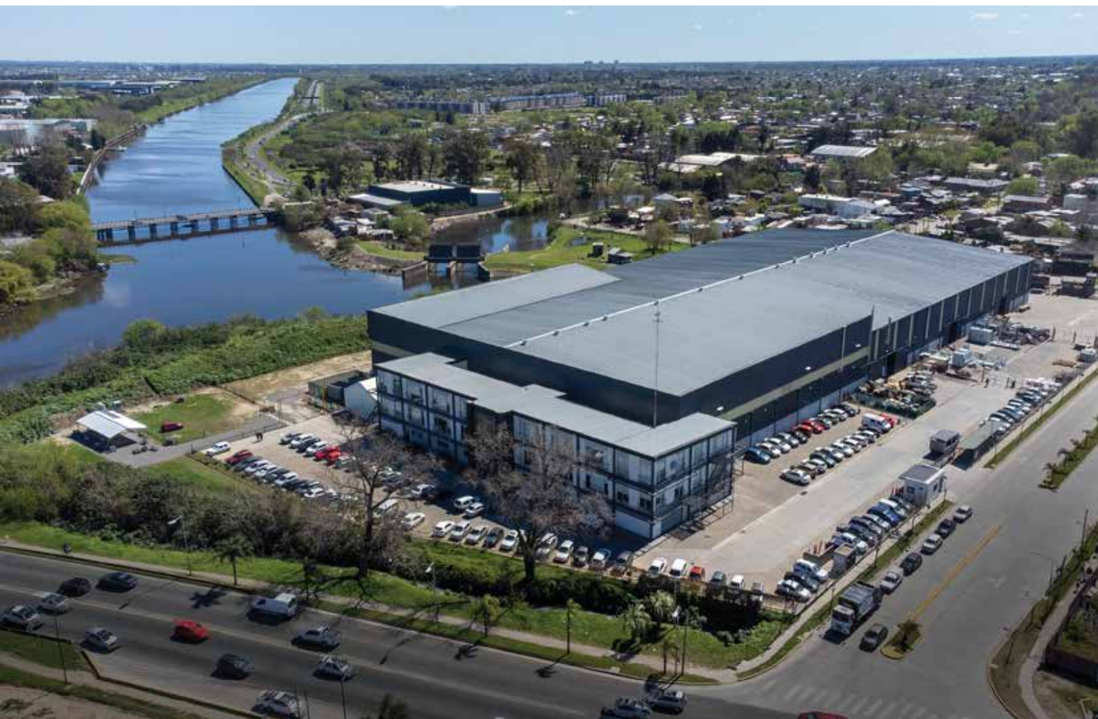
Aspro industrial plant
